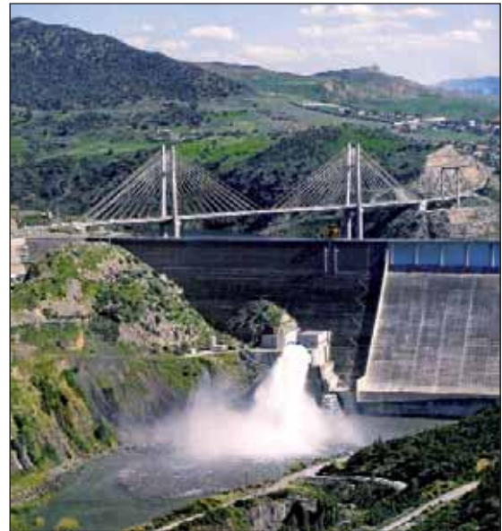
View of Beni Haroun, Algeria's largest dam.
